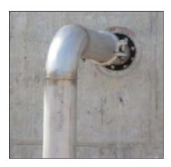
Many of these applications involve connections where the pipe is penetrating a wall, floor or ceiling and sealability is required between the pipe and the penetrated surface. Through wall applications are an area where a mechanical seal needs to be utilized in order to reach complete sealability.
